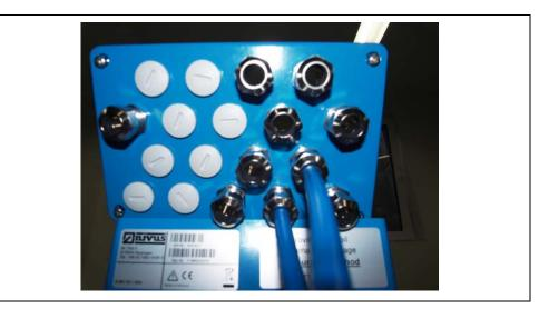
Fig. 5-26 Inserted sensor cable - exterior view path 1
